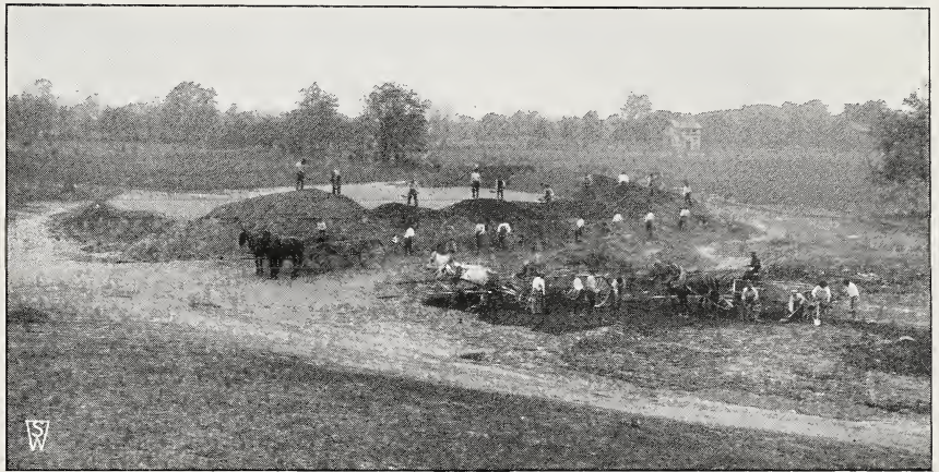
Constructing one of the greens at the Nassau Country Club, L. I. Stumpp & Walter Co.'s seeds were used on this course
